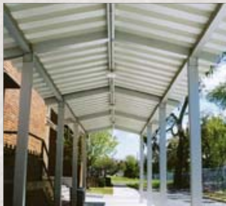
Metal Walkway Canopy
