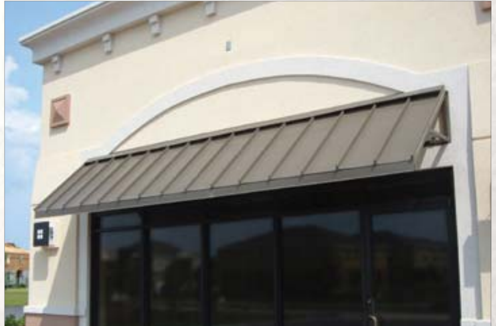
Bahama Style Metal Awning
