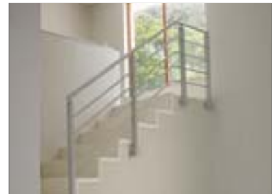
Interior Custom Handrail
