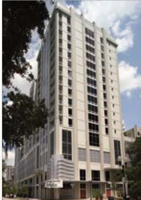
The Paramount on Lake Eola Orlando, FL Perforated Metal Wall Panels
