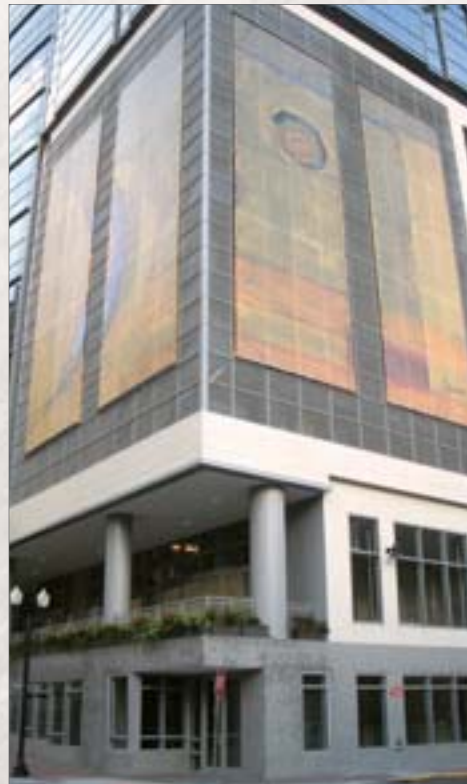
DyneTech Centre Orlando, FL - Fabric Wall Panels
