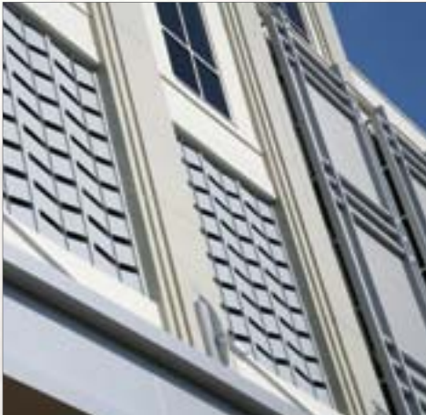
The Paramount on Lake Eola Orlando, FL Perforated Metal Wall Panels & Metal Mesh Wall Panels
