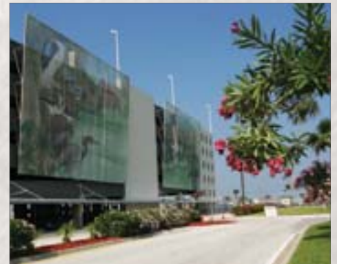
Port Canaveral , FL - Fabric Wall Panels
