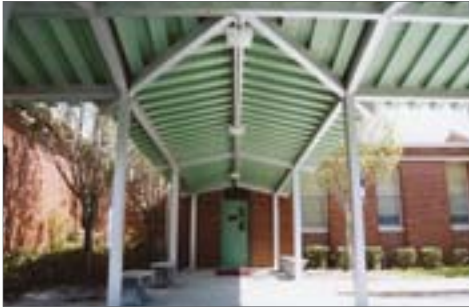
Metal Walkway Canopy
